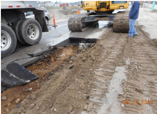
Trench Preparation for new Sewer Installation
