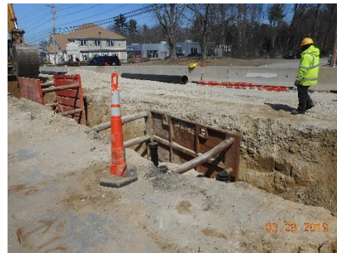
New Water Main Installation
