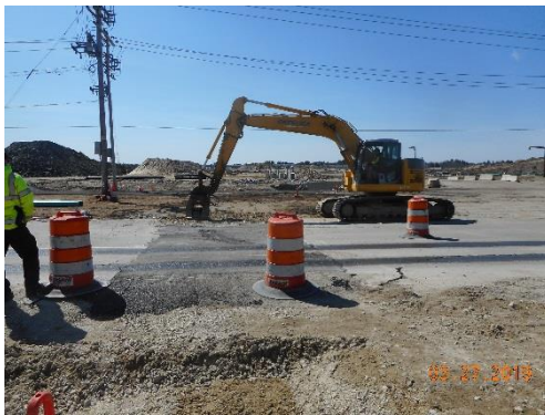
Sewer Trench Excavation
