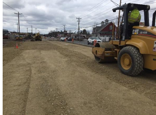
Paving preparation near the bridge
