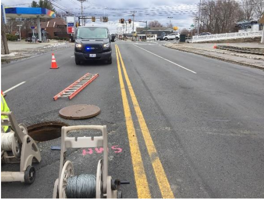
Sewer Testing along South Broadway
