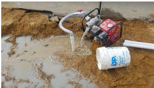
Groundwater Wellpoint Test and Clearing
