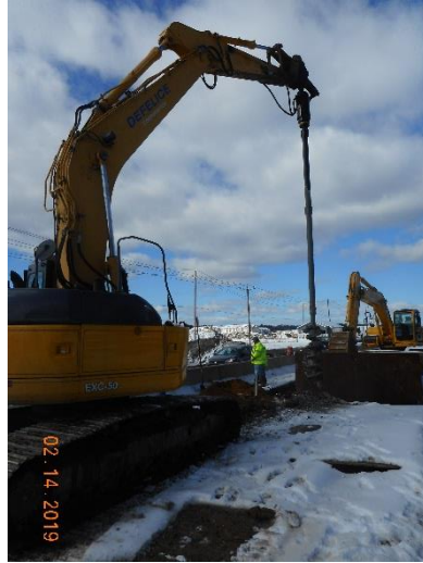
Dewatering Wellpoint Install
