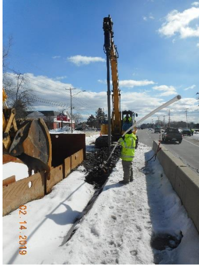
Dewatering Wellpoint Install
