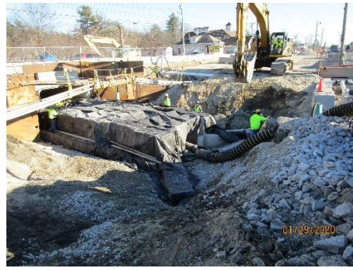
Temperature controlled tent for Curing
