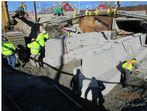
Footing Installation for Bridge.
