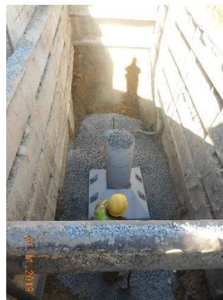
Sewer Chimney Structure Installation
