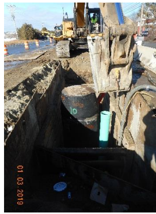
Sewer Manhole Installation
