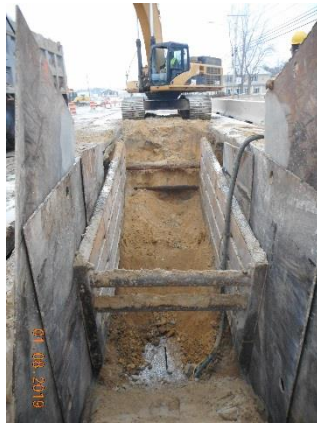
Sewer Trench Excavation
