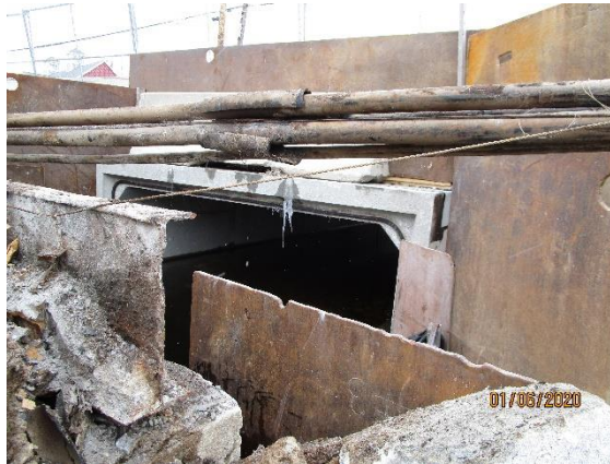
Concrete banks around telecommunication ducts removed
