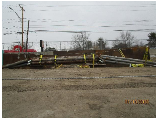
Telecommunication Ducts suspended to allow bridge installation underneath
