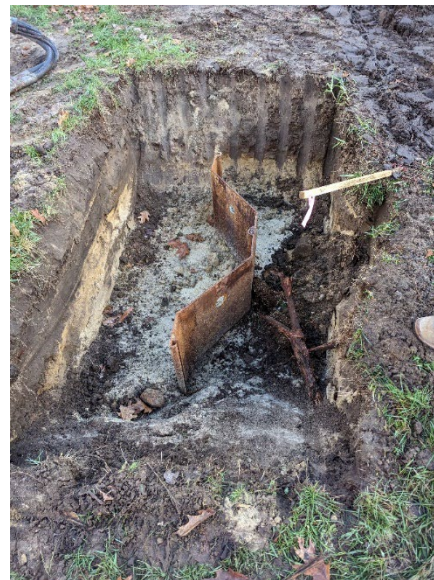
Pile head trench, with electrode pile installed.
