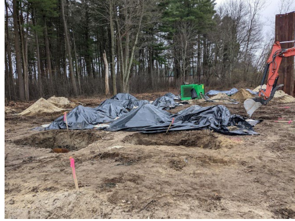
Open channel pile head trenches and stockpiles.
