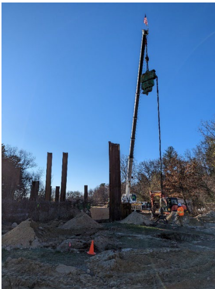
Crane preparing to drive electrode pile.
