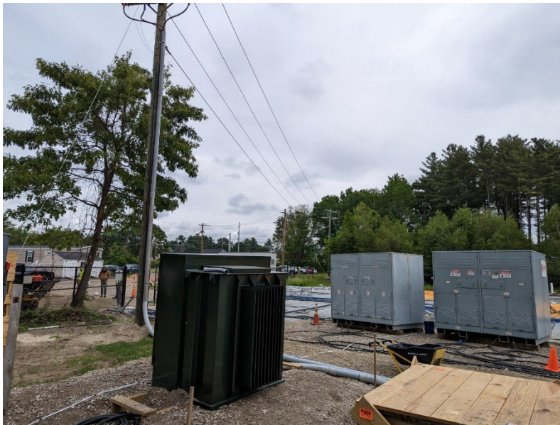
Newly installed electrical poles and step-down transformers.
