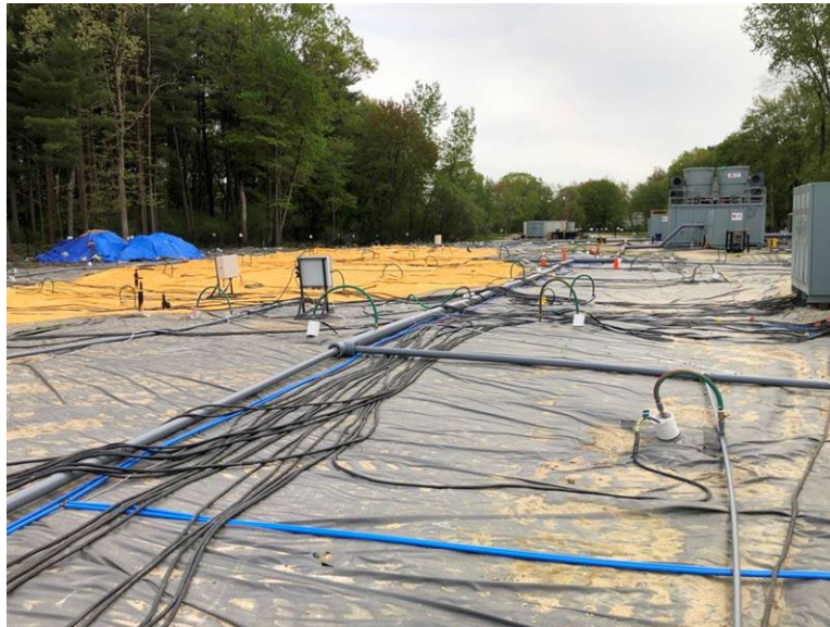
Ground view of the completed liner, power cables, and pile heads.
