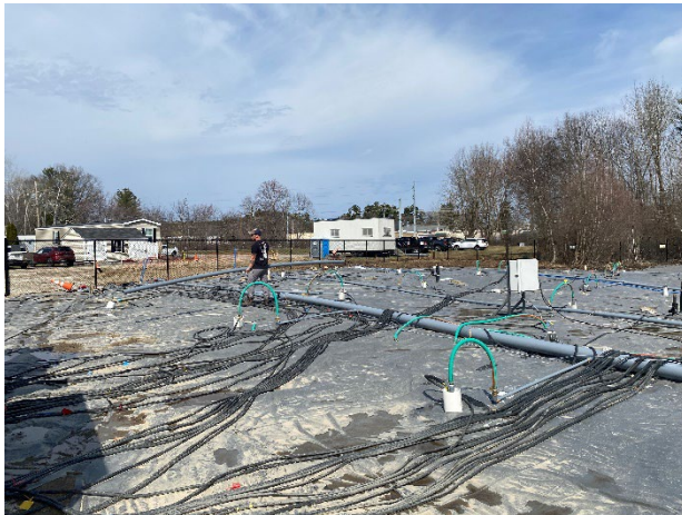
Electrical cables and vapor hose connections.
