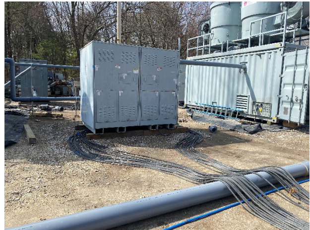
Electrical cable connections to transformer.
