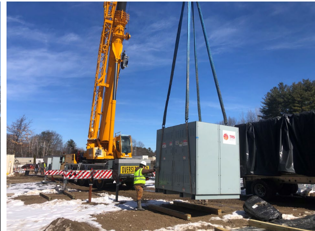
Delivery and crane unloading of electrical transformers.
