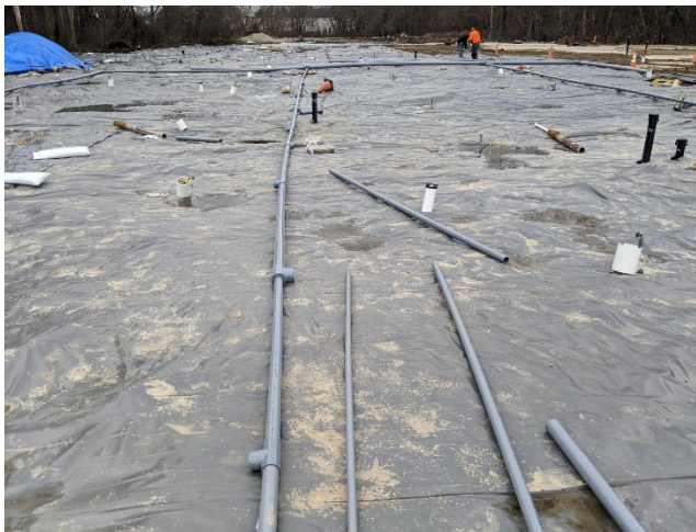
Vapor recovery piping construction
