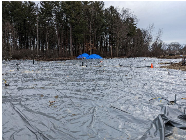
Installing the ground covering liner.
