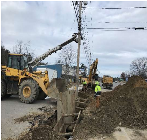
Utility Pole being Held to Install Pipe
