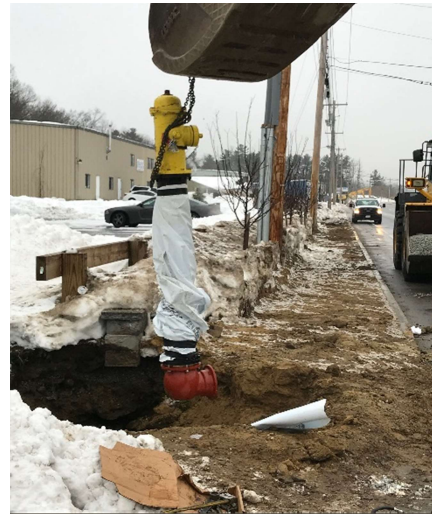
Hydrant Installation along Route 28
