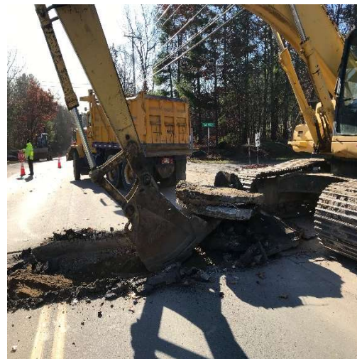
Preparation for Water Main at a Road Crossing
