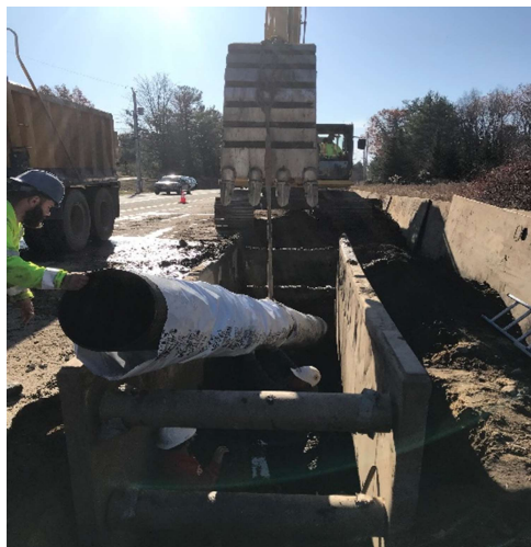
Water Main Installation
