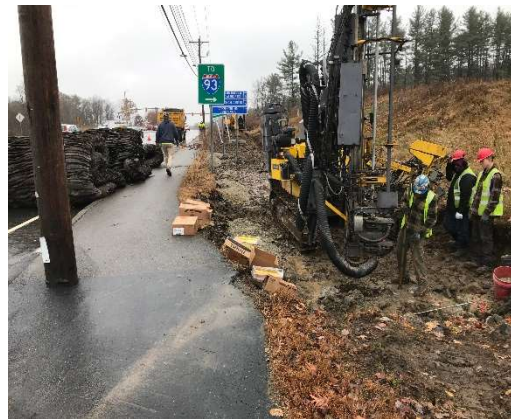
Drilling and Blasting Preparation
