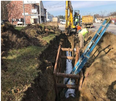
Water Main Installation along Route 28
