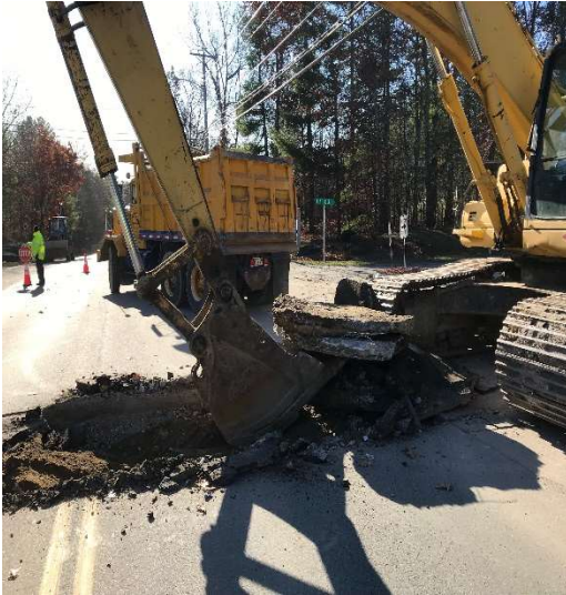
Preparation for Water Main at a Road Crossing
