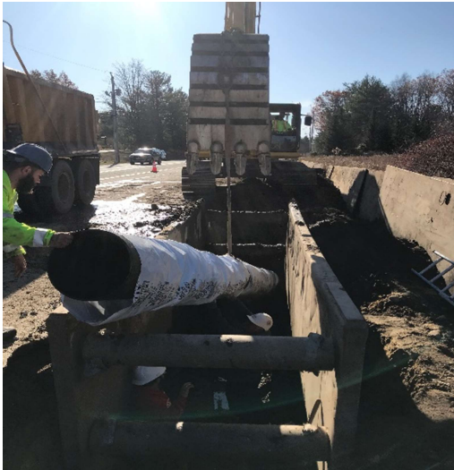
Water Main Installation
