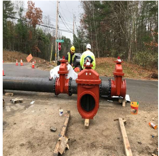
Water Main Gate Valves Installation
