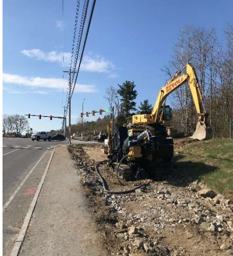
Directional Drilling Begins at Route 111
