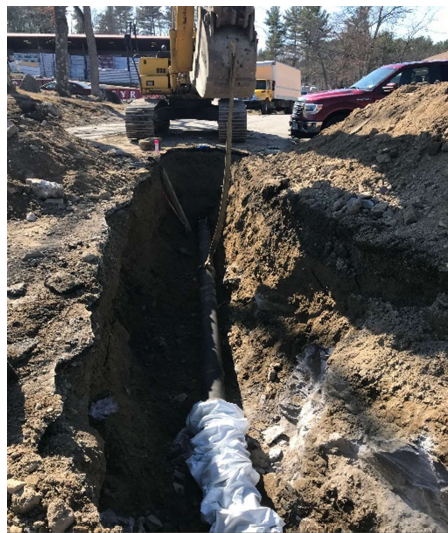
Water Main Installation
