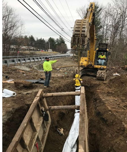
Fire Hydrant Installation
