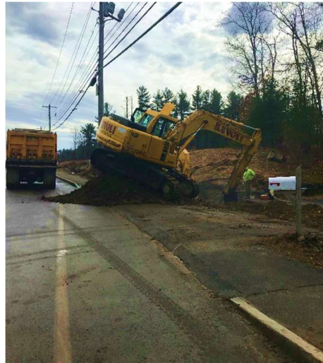
Excavator Crushing Ledge for Water Main Trench
