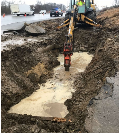
Digging a Water Main Trench
