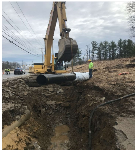
Water Main Installation
