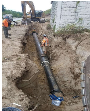
Water Main Install under Pedestrian Bridge
