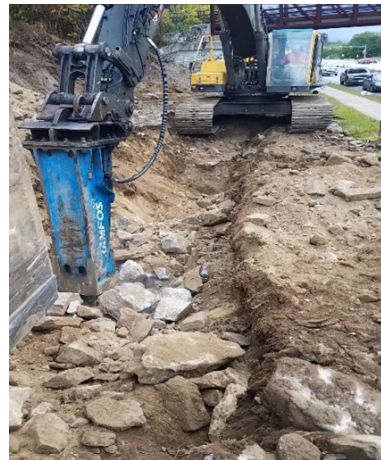
Hydraulic Hammer Crushes Rock
