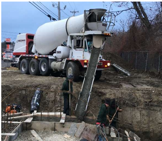
Concrete Pour for Foundation Walls at Rail Trail
