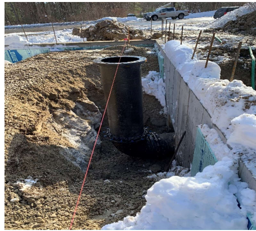
Pipe Assembly Installation at Northland Road
