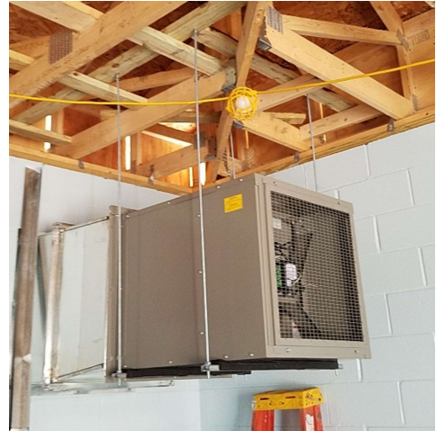
Exhaust Fan Installation at Rail Trail
