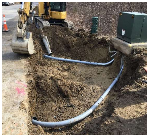
Tie-in to Northland Road Transformer
