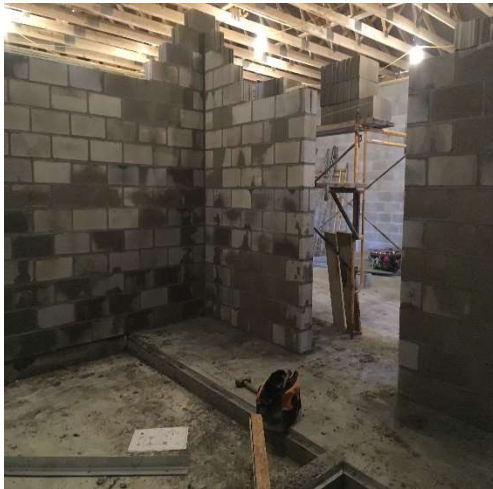
Interior CMU Block Being Placed at Northland
