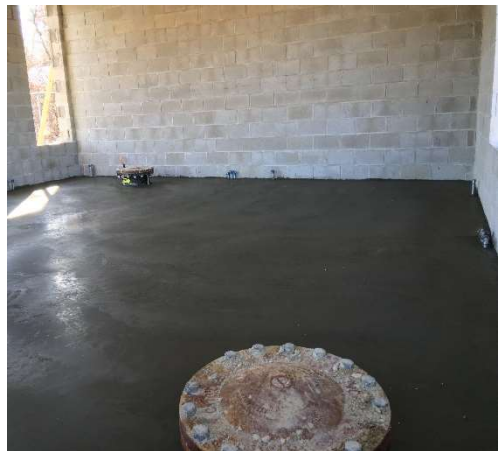
Concrete Slab-on-grade at Rail Trail
