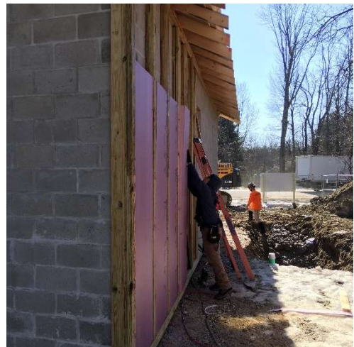
Siding System Being Installed at Northland
