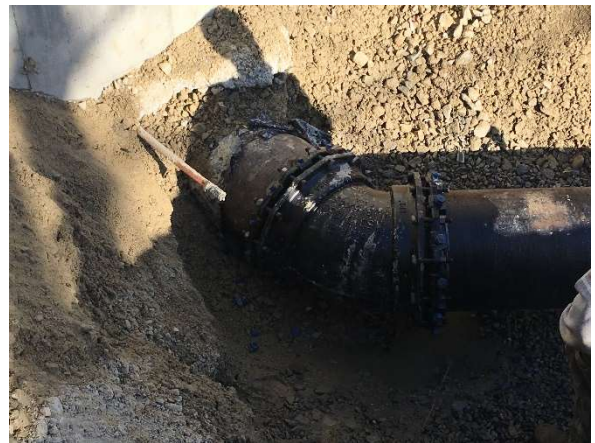
DI Pipe and Bends Installed at Rail Trail
