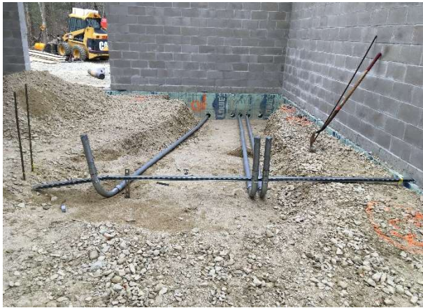
Three Electrical Conduits Installed at Northland
