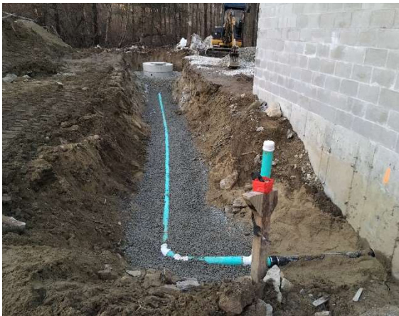
Drain Pipe being Installed at Northland Rd
