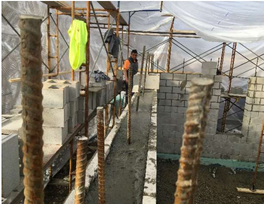
Reinforcing Bars in the Walls at Rail Trail
