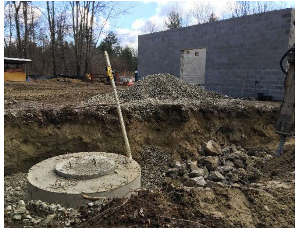
Dry Well Installation at Northland Road
