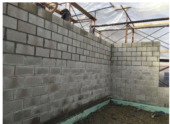
Erecting Masonry Block Walls at Rail Trail
